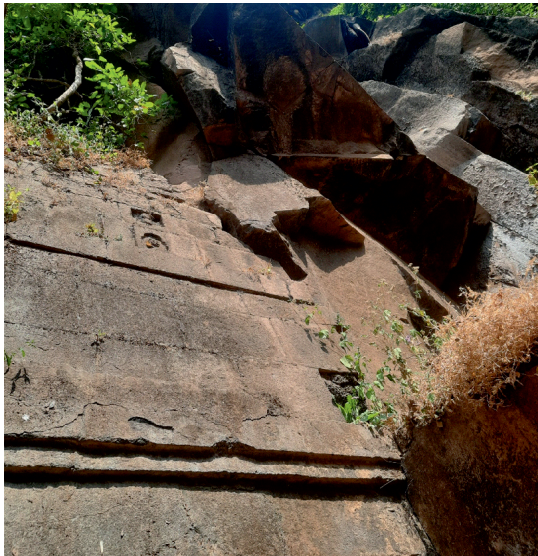
Figure 3: Masonry stone blocks at the façade
